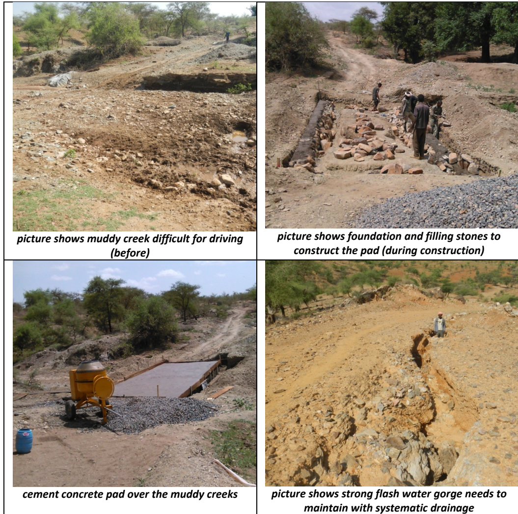
Figure 18.12 Road Maintenance Along the Road to the Mato Bula Deposit
