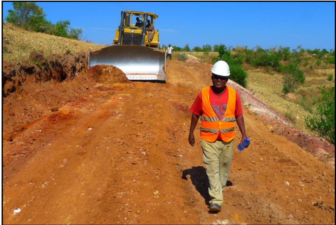
Figure 9.1 Reverse Circulation Drill Line Being Prepared Using the Dozer at the Terakimti Deposit
