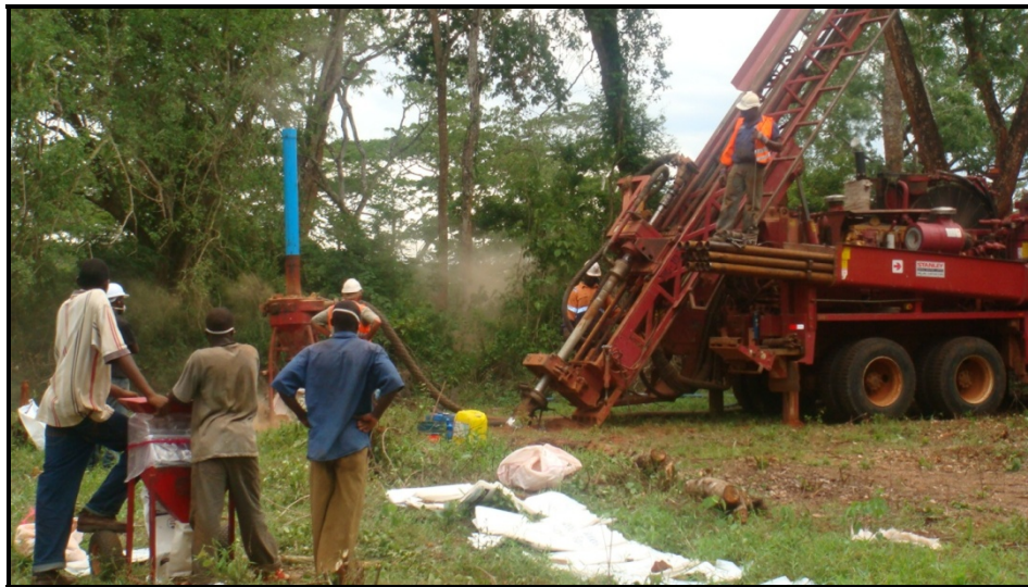
Plate 7. Reverse circulation drilling, Semwaliko area (archival photo)
